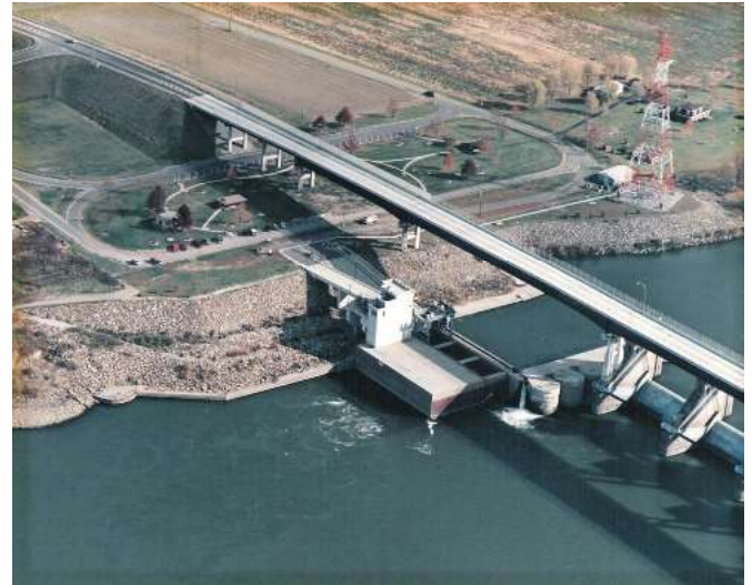
Greenup Hydro Plant (AMP & Hamilton owned) Estimated Capacity = 70.2 MW Commercial Operation = May 1982
